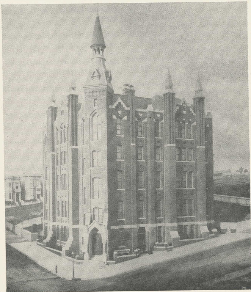
Cooper Medical College. Original building, ca. 1882.
